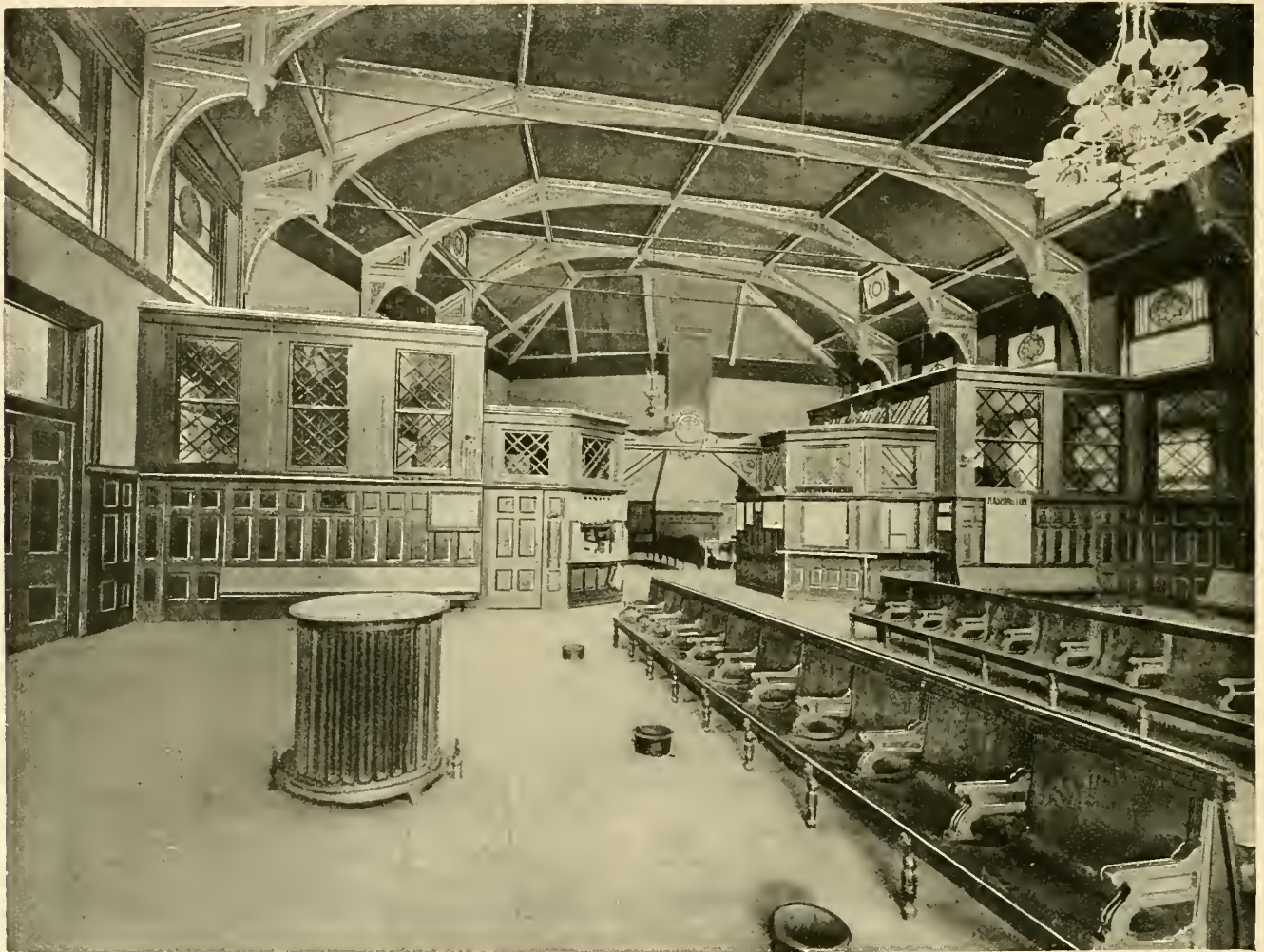
INTERIOR VIEW OF MARKET STREET STATION, PENNSYLVANIA RAILROAD.
